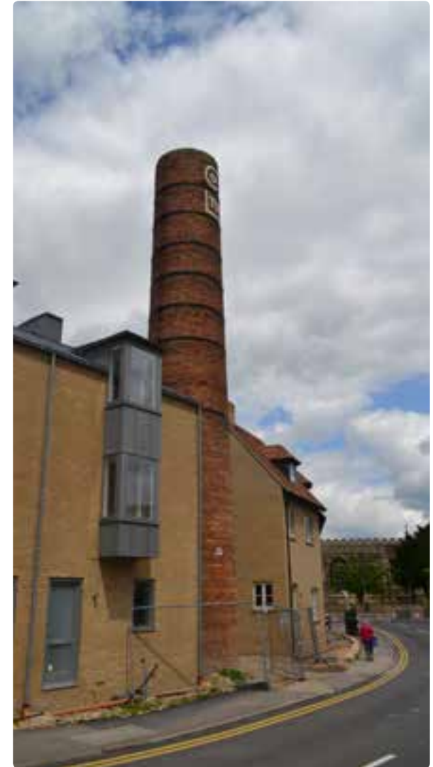
Retention of chimney in new development
