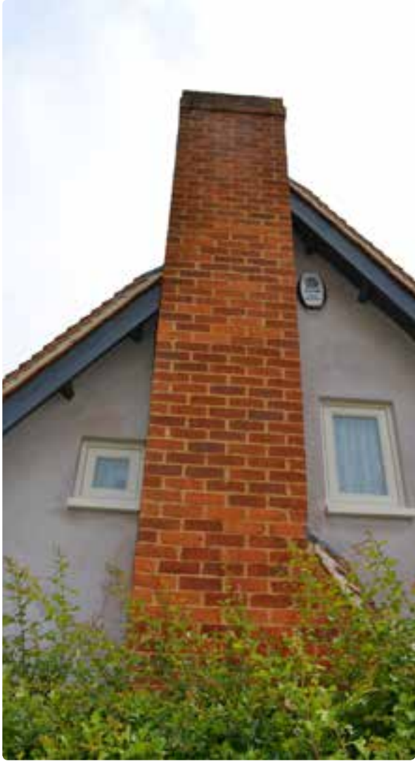
exposed brick chimney, variation in windows and exposed timber verge details
