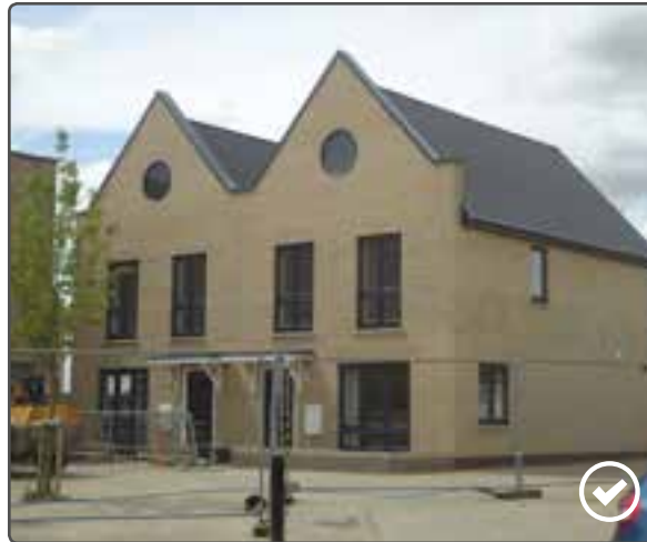
Successful use of materials and window to gable, Bydand Lane
