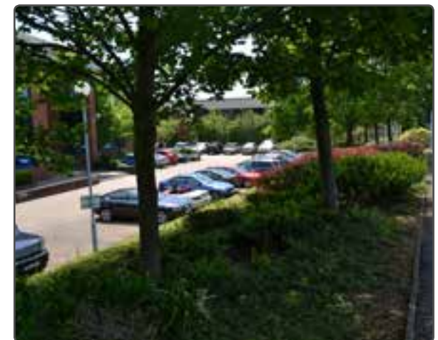
Office building set back from the street to allow some car parking to the front
