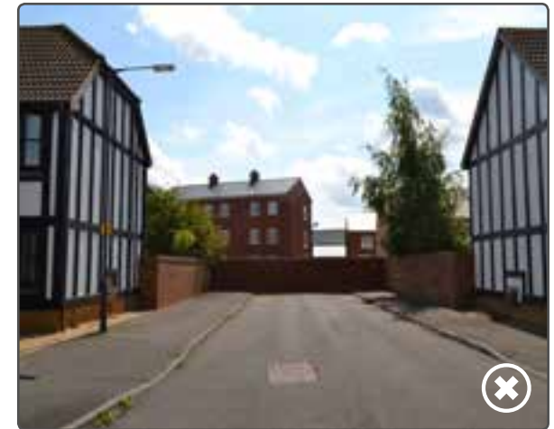
This is very poor. These two developments have been separated by a brick wall! - Bedford
