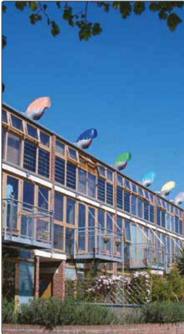
The amount of glazing on this building maximise the natural light into it
