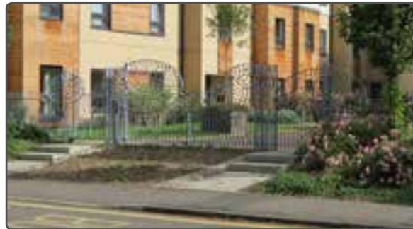
Railings and gates fronting Brookside, Huntingdon
