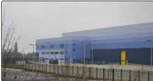
Colour banding helps to blend the building into the landscape
