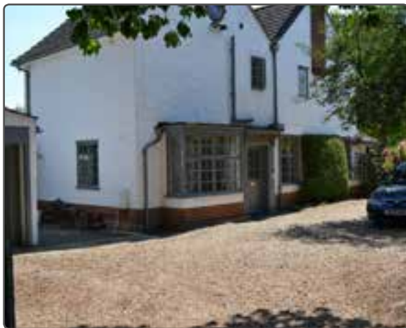
The size and the colour of the bay window creates additional interest
