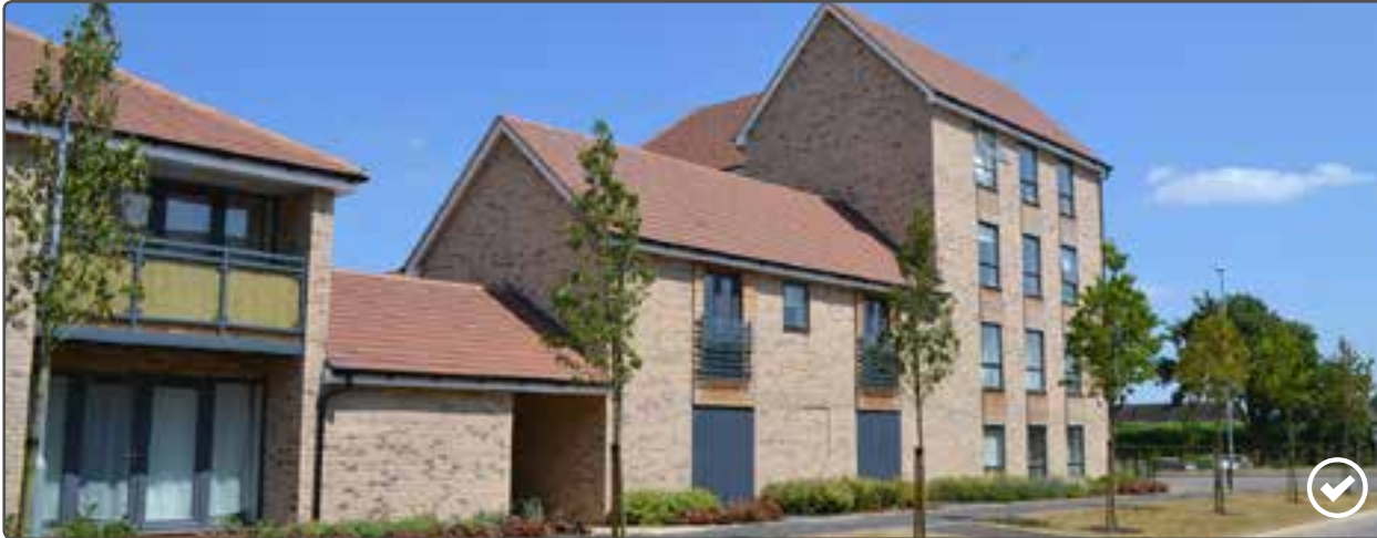
This is good example - the single storey bin store has been incorporated into the building
