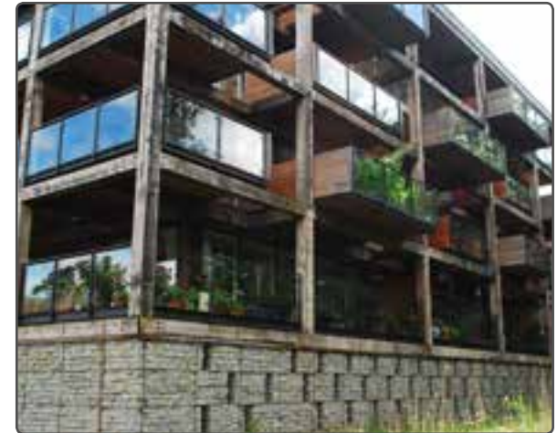
This building uses semi basement parking behind gabions that are designed to let natural light in
