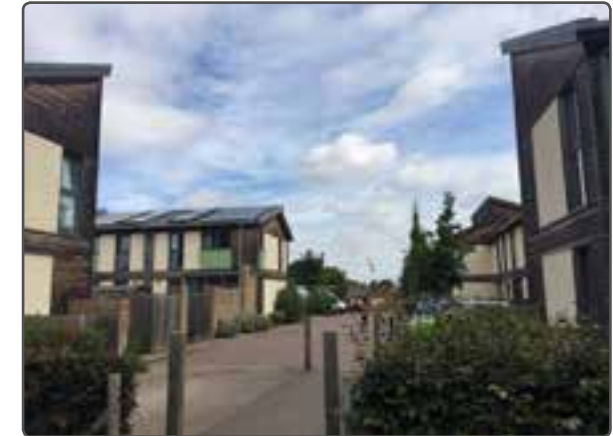
Staggered first floor windows to avoid direct overlooking
