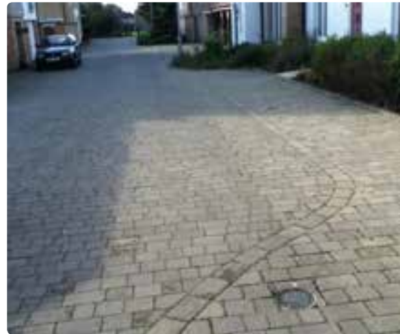
High quality paving materials
