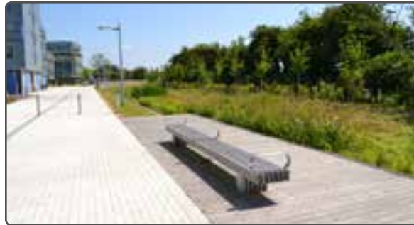
Drainage channel following pedestrian route
