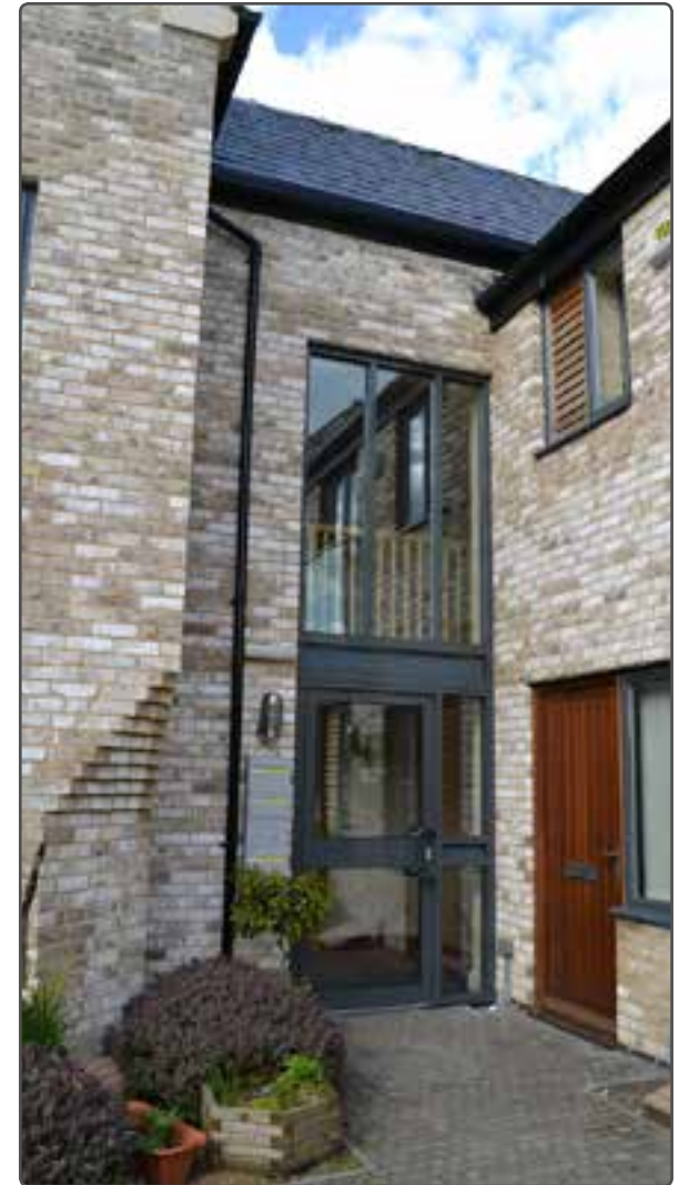
Pleasing shared entrance design to flats
