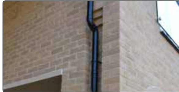
Carefully disguised pipework - Huntingdon
