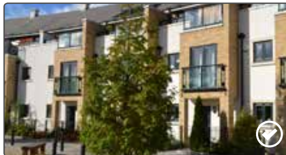
Top floor external balcony
