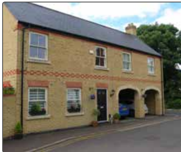
Slate roof at Temple Close, Huntingdon
