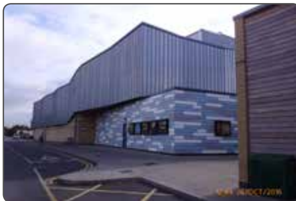
Scale and mass of the cinema building broken up through use of subtle variation in height, undulation on external cladding and different use of materials and colours, Rowley Arts Centre, St Neots
