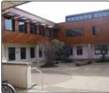
Office building central space
