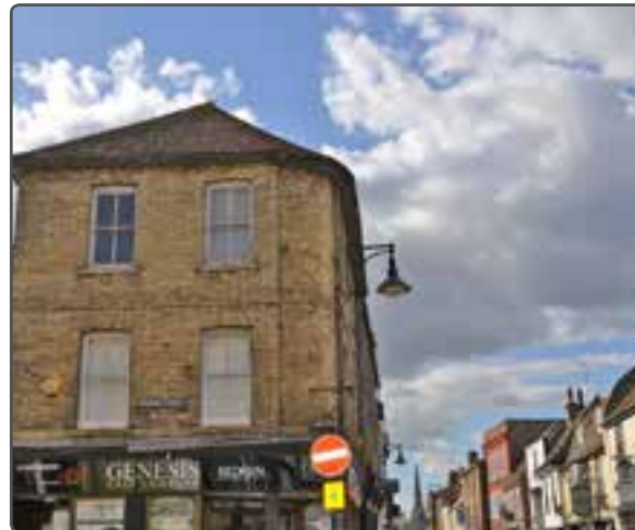
Street light attached to building to reduce clutter
