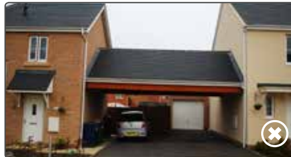
This is a poor example of where a poorly proportioned car port structure detracts from the wider street scene
