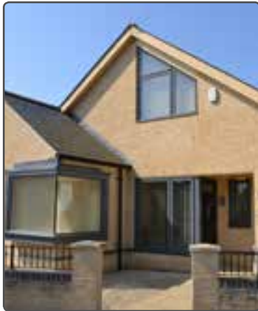
The interplay between windows set in a reveal and boxed windows is appealing here
