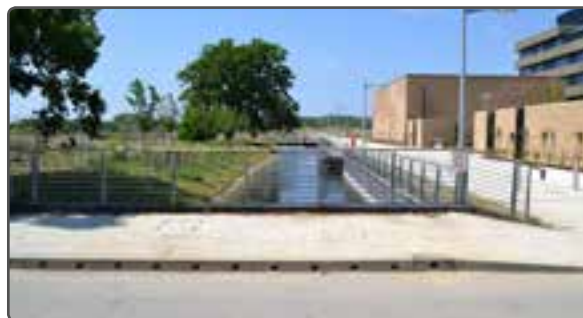
The stream is canalised at this point
