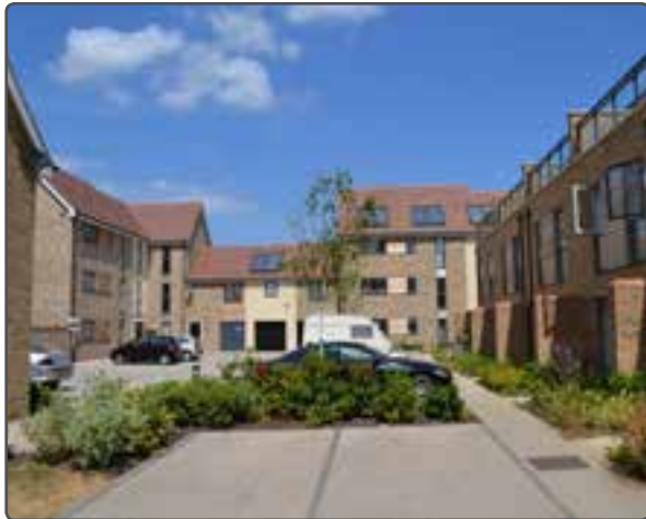
Car parking court well overlooked by properties and including lots of soft landscaping
