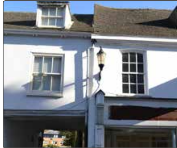
Street light in a good location
