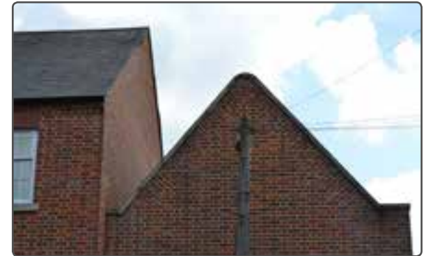
Tumbled brickwork
