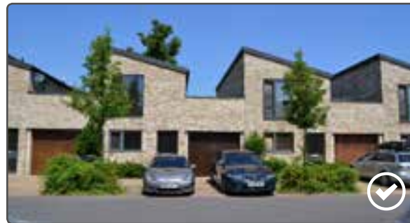
On plot car parking can work well when accompanied with robust and well designed soft landscaping - Cambridge
