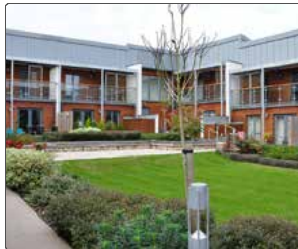
Well landscaped courtyard space
