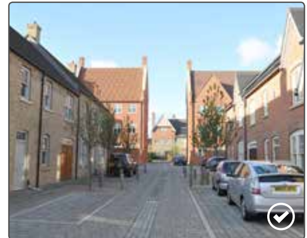
In this high density area car parking spaces are identified by the use of different materials
