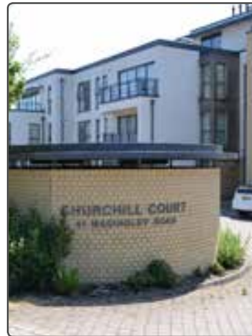
Well ventilated bin store
