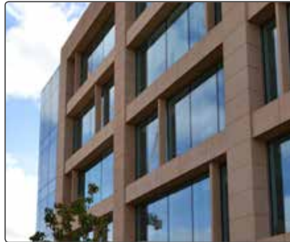
Deep reveal on this office building
