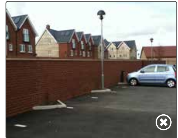
How not to design a car parking area - a harsh place, with no breathing space for any landscaping
