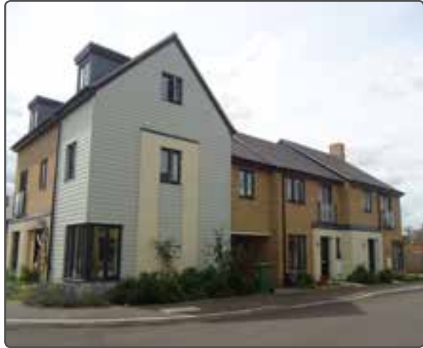
Corner of development block with changes in scale and design - Little Paxton
