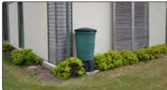
Water butt - rainwater harvesting
