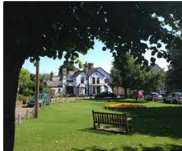
Focal building at the northern side
