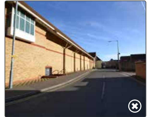
This service road is overengineered and not pedestrian friendly
