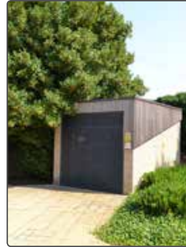
Substation clad in contemporary design
