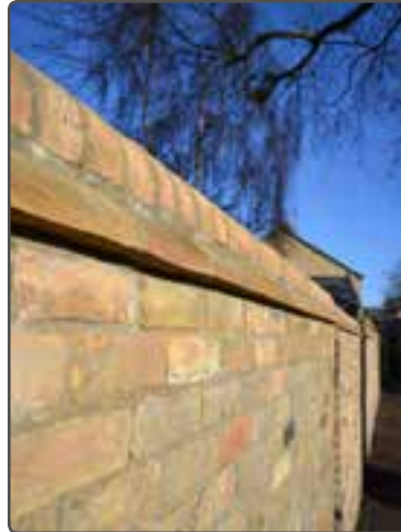
Well detailed brick wall
