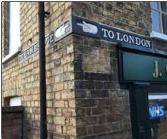
Direction sign attached to building
