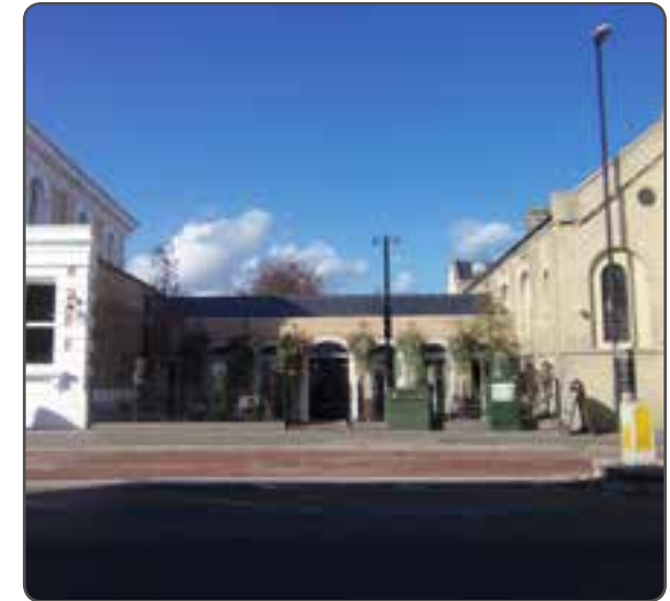
View of extension from George Street
