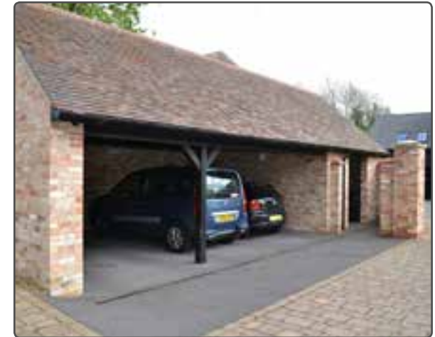
This same development in Brampton uses a car port structure that is well proportioned and uses high quality materials. It is also used as a cycle and bin store.
