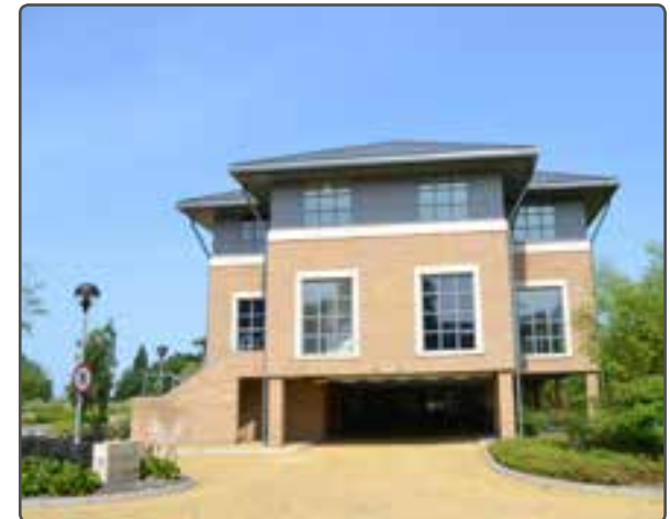
This office building has undercroft parking that is well lit by natural light
