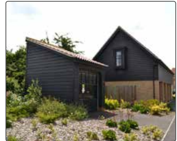
Substation design reflecting adjacent building
