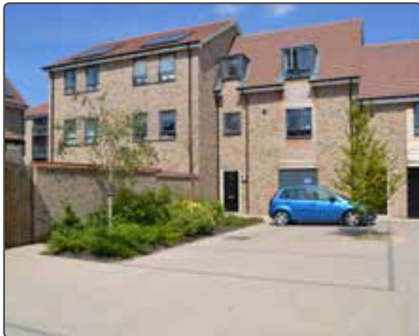
This car court is broken up with some attractive areas of landscaping and delineation of parking bays
