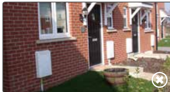
Poorly located meter boxes - St Ives
