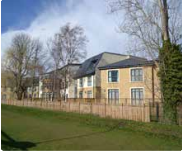
Use of large windows
