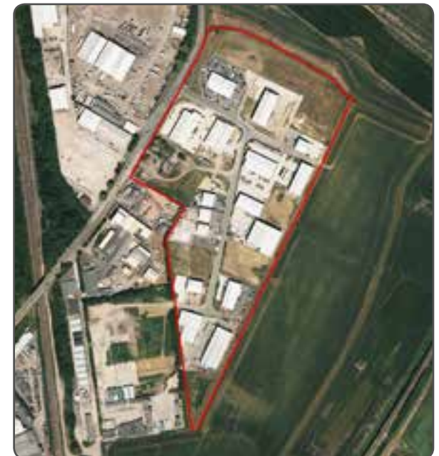
Aerial view of Eagle Business Park, Yaxley
