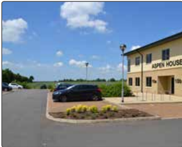
Setting the car parking away from the office building helps to create a pleasant working environment - Huntingdon
